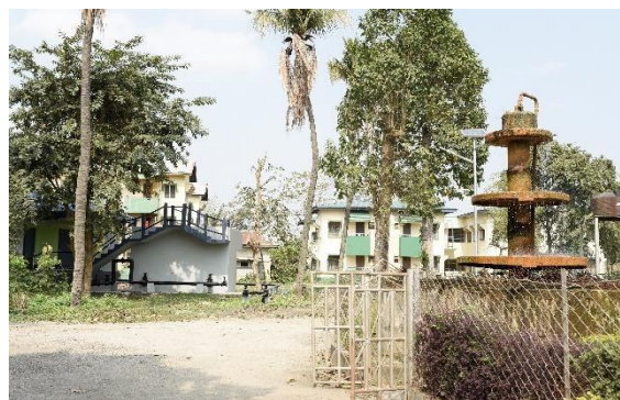
Figure 2. 12. Water treatment plant
