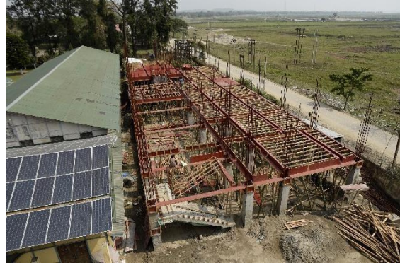
Figure 2. 14. New Laboratory building under construction
